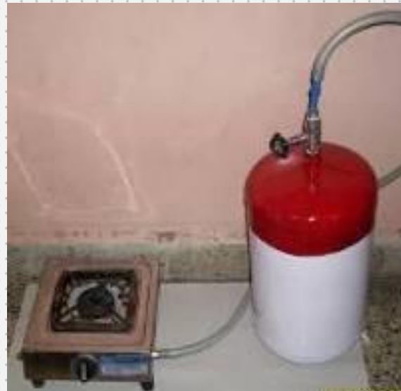
Upgraded and bottled biogas for use as a cooking fuel
