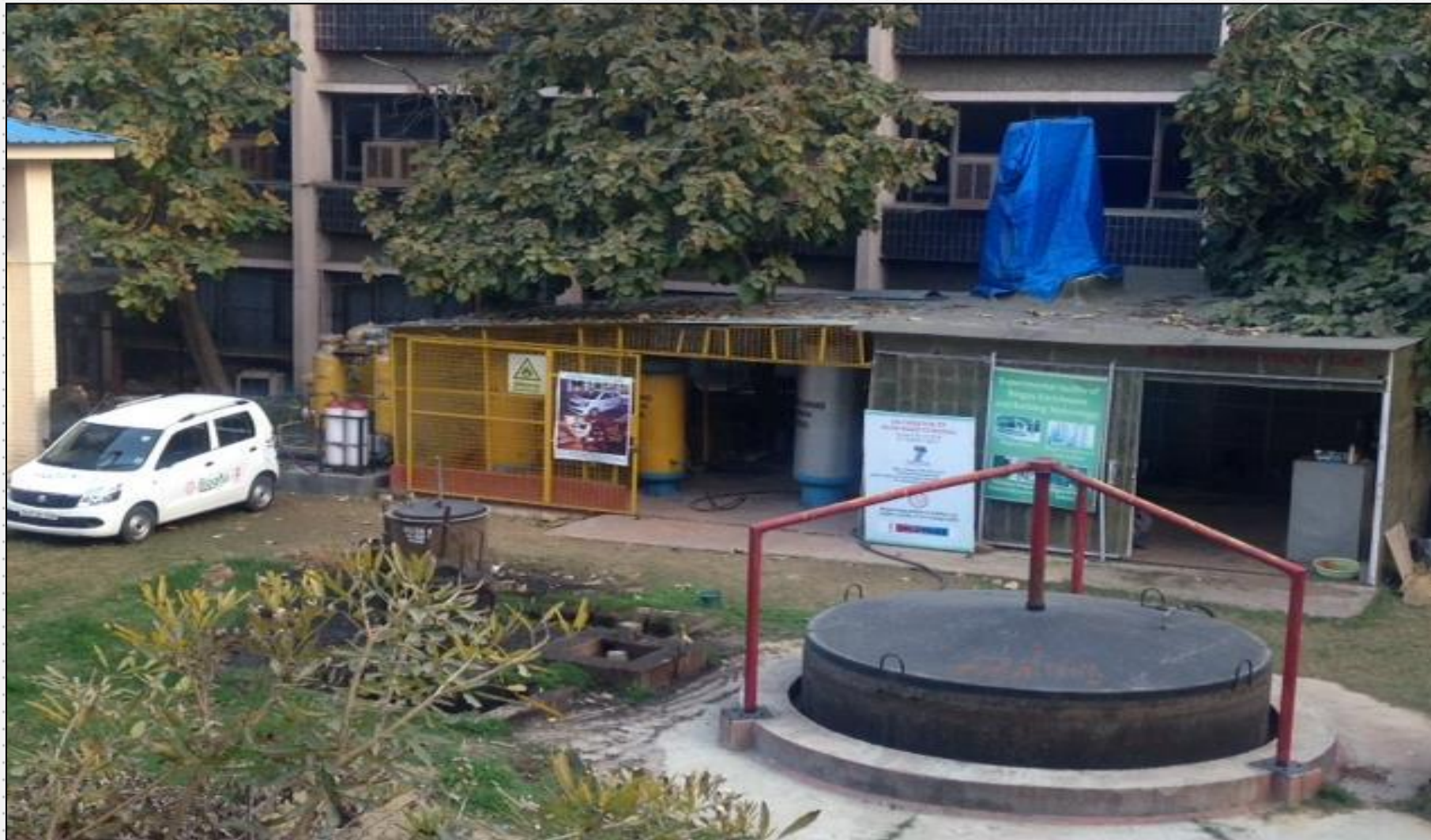
Water Scrubbing based BioCH 4 and BioCO 2 Production System at IIT Delhi
